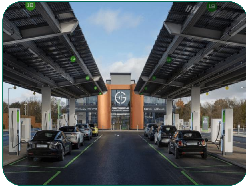
Dec 2020: Gridserve opened the UK's first electric forecourt
